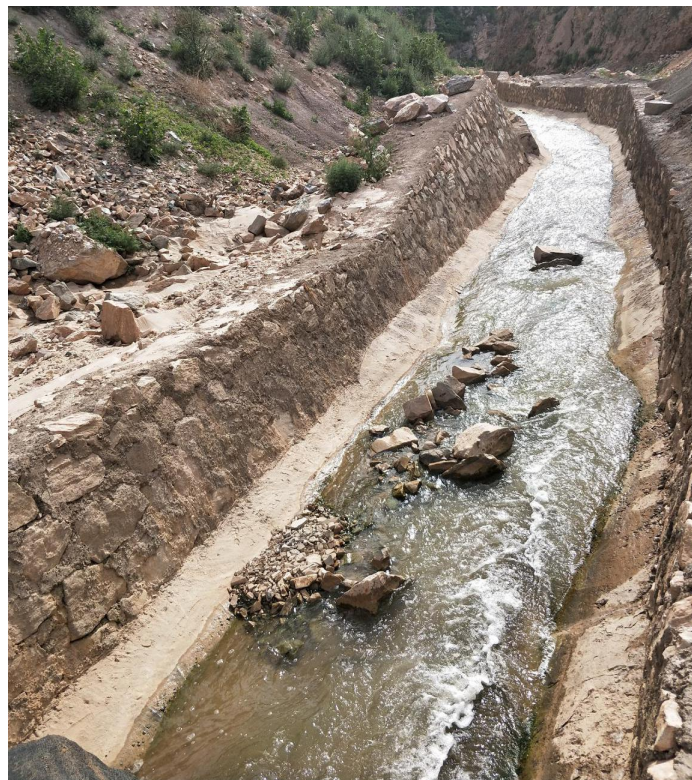
磨石峡河道修缮
